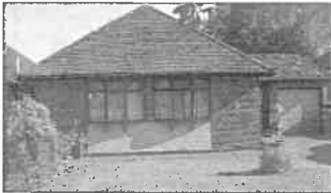
The Done house
